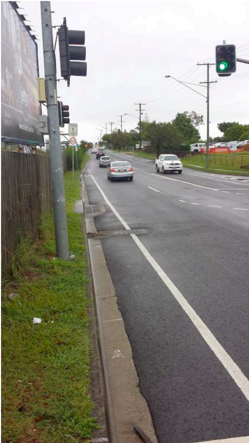
Bridge Street, Albion. A “bike lane” becoming a “bicycle awareness zone” in a 60 km/h zone.
