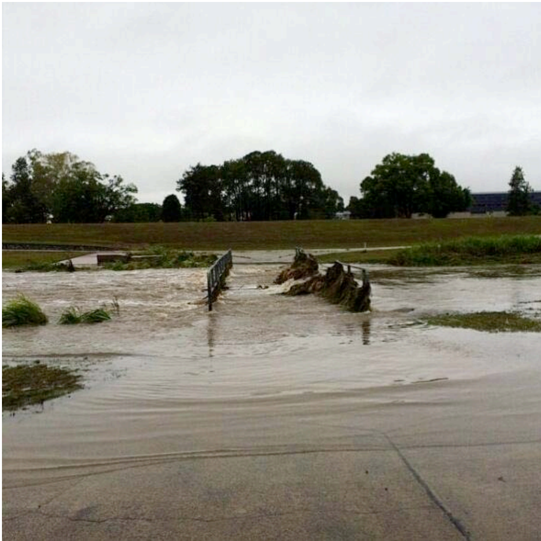
Kedron Brook Bikeway, March 2014 after rain. Much of Brisbane's dedicated bikeway network is built on floodways. 29
